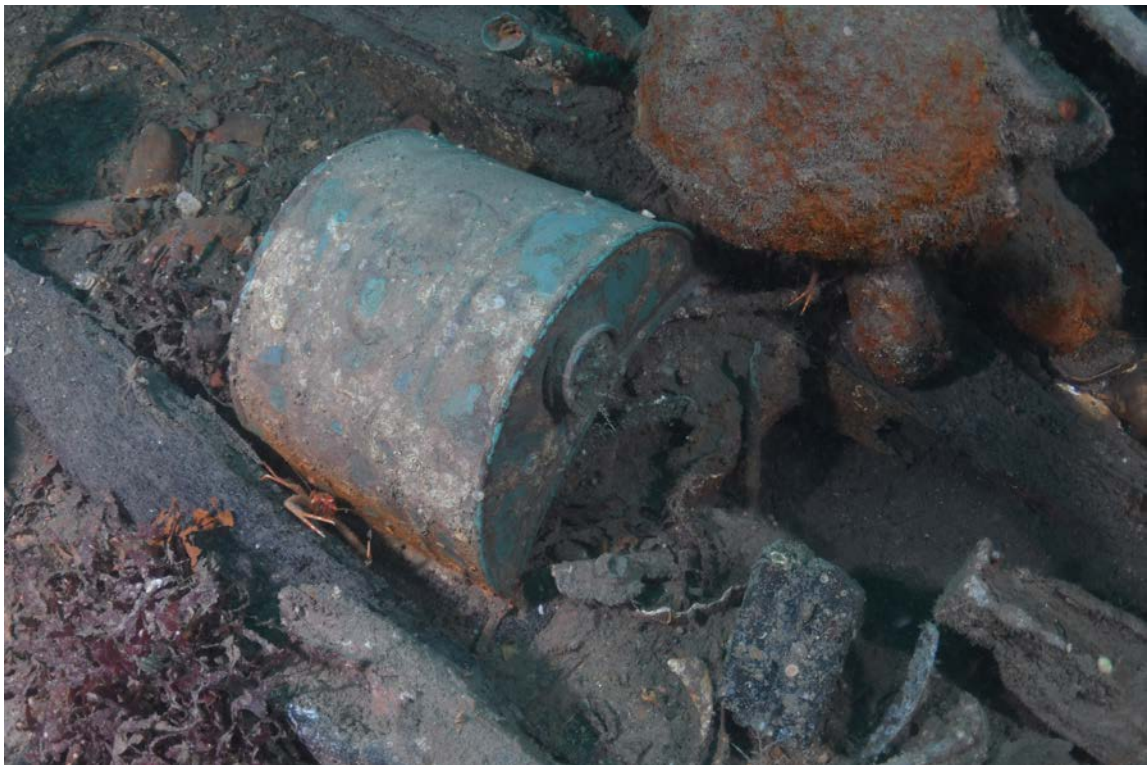
Figure 23: Copper saddle tank among boiler pipework.
